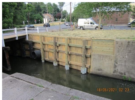
Newly Completed Repairs to Canal at Bridge
