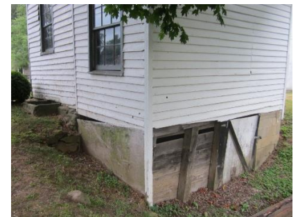
TOLL HOUSE FOUNDATION
