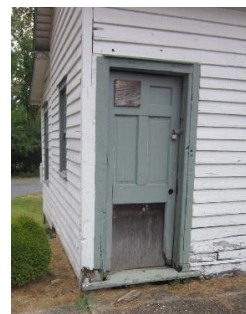
TOLL HOUSE DOOR
