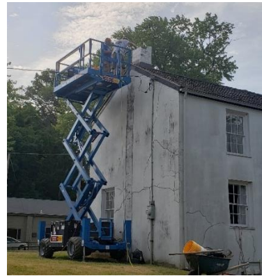
WORKING ON TH NORTH CHIMNEY
