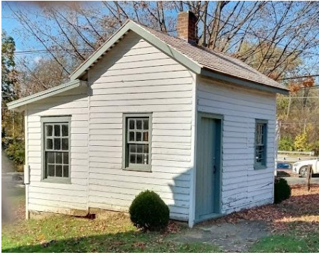
TOLL HOUSE with new door and roof
